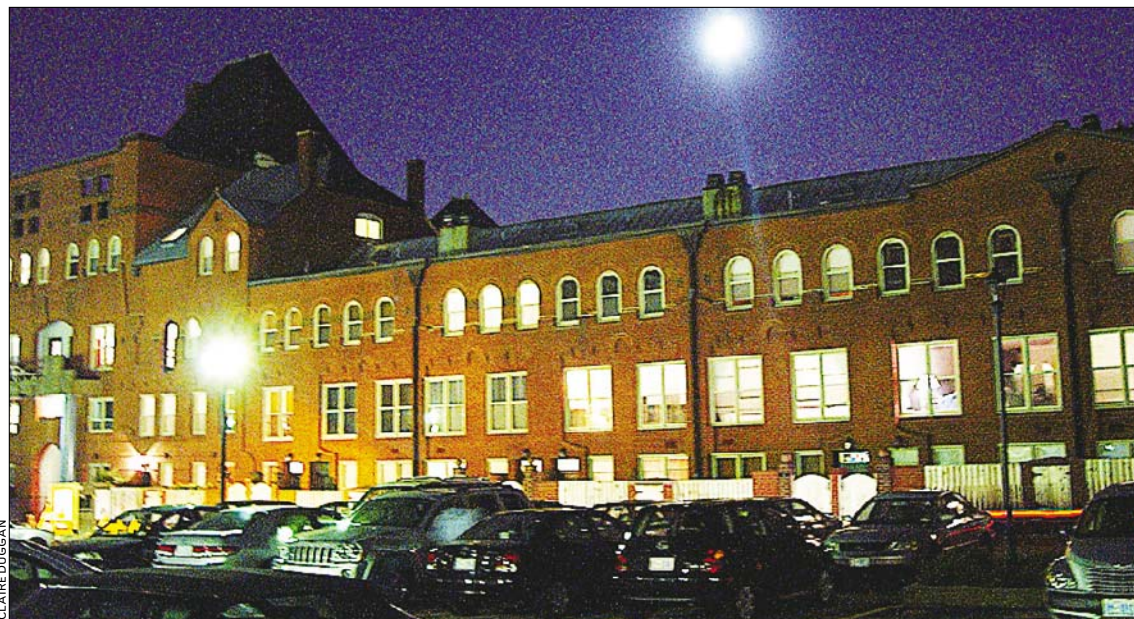
CONVERTIBLE: Developers maintained much of the original character when converting a streetcar depot into the Car Barn.
